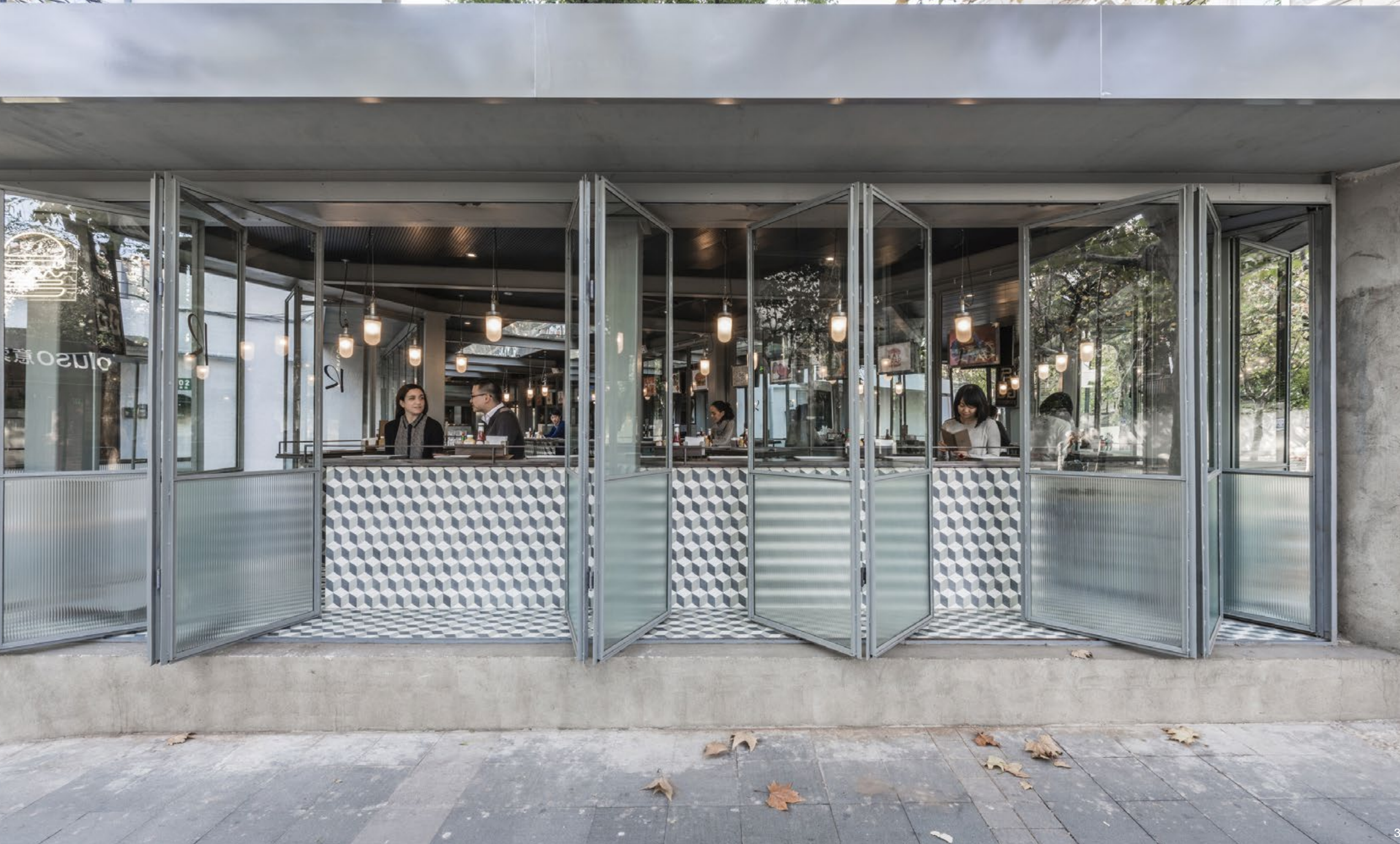
3. 設計師運用玻璃的通透特性，打造出數十片摺疊門作為店面外觀。4.5. 摺疊門以清玻璃與具有紋理的結構玻璃打造而成，供業主隨天氣情況自由決定開放範圍。6. 明亮的日光與悠閒的武康街景穿越了玻璃門面、引入室內空間。7. 摺疊門以金屬鑲形，在開關時呈現出立體的曲折結構。 3. Glass folding doors set a total transparent facade 4.5. Folding doors provide flexibility to give access between inside and outside 6. Natural light permeates inside to give a tranquil impression 7. Folded door exhibits a special sculpturing profile
