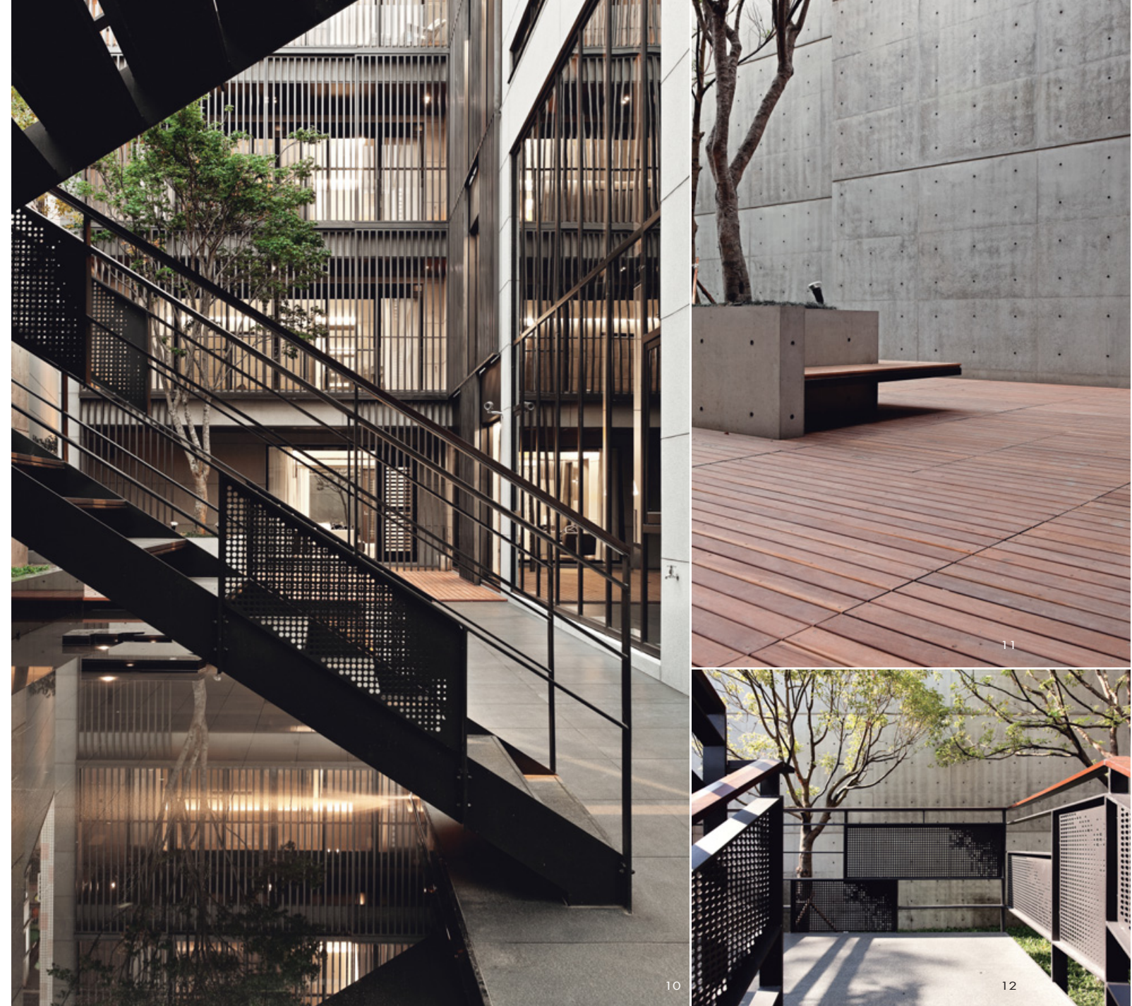
9. 純粹而精練的建築手法，使得整個空間呈現出一種靜謐的姿態。10. 經由一座戶外樓梯通往半戶外空間。可與南台灣的氣候產生互動。11. 戶外庭院。12. 樓梯扶手以點狀沖孔板製造漸層效果，呼應樹葉搖曳的動態感。 9. Building and interior have an integrated link 10. Staircase leading towards a terrace 11. Outdoor courtyard 12. Handrail details of the staircase - perforated boards allow light to pass
