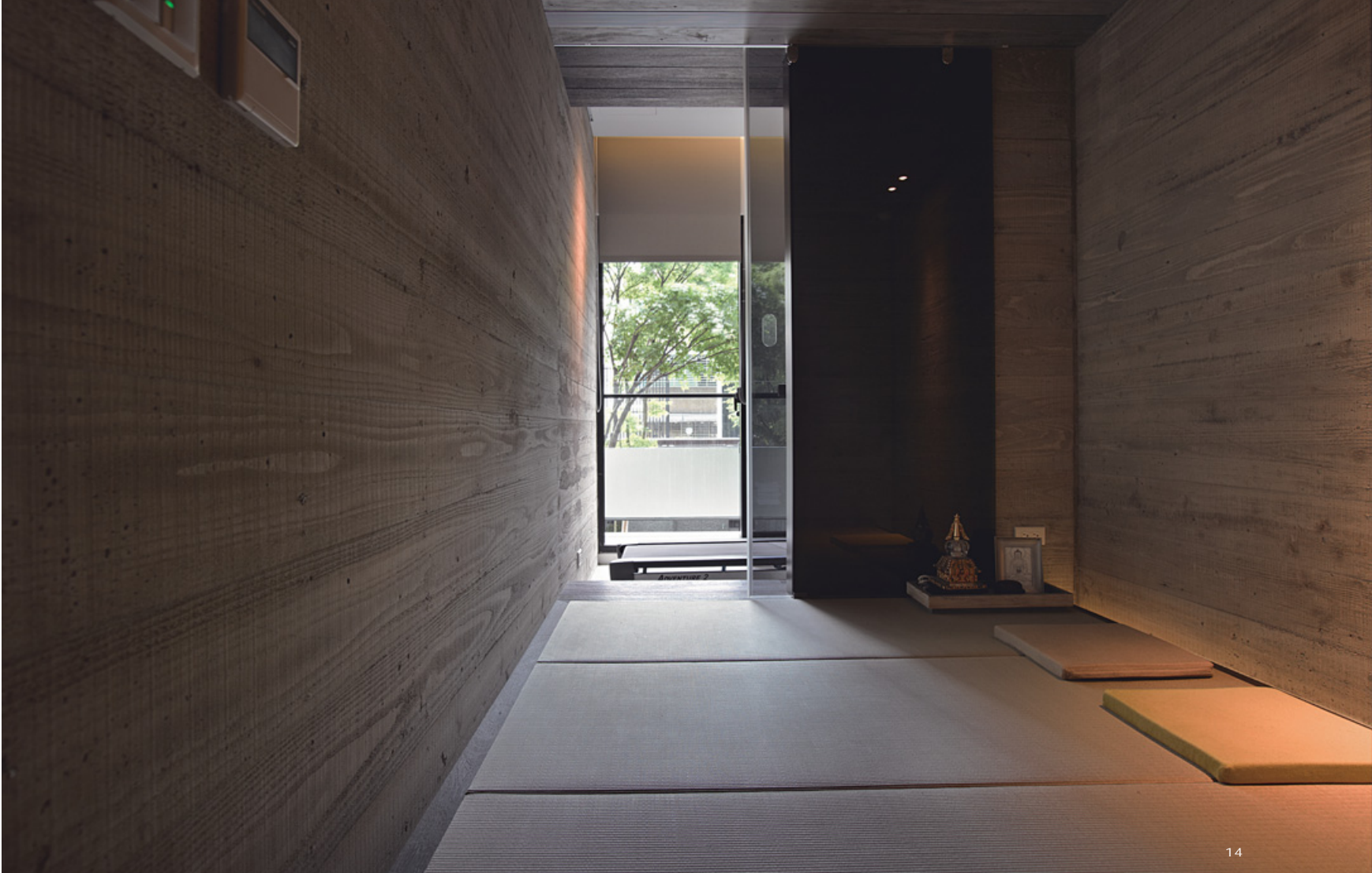
14. 禪房燈光以地照式照明呈現，強化靜謐感。15. 禪房的兩道主牆以清水模灌模而成。 14. Zen room and its lighting quality 15. Zen room and its two exposed concrete walls
